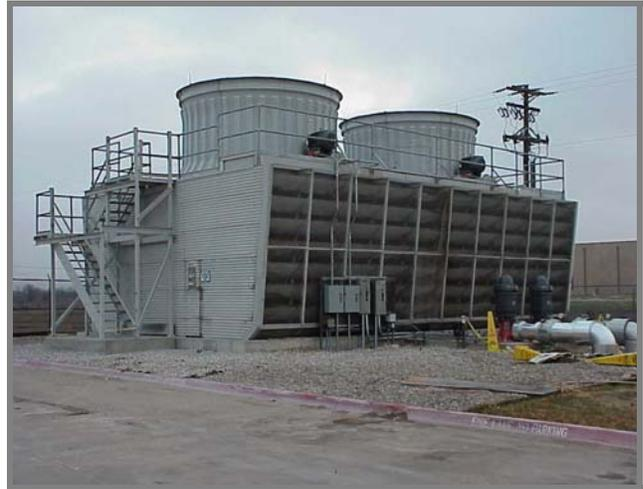
A bulk-mail handling center in a Dallas suburb has almost 800 thousand square feet (74,300 square meters) of mail processing area. Air conditioning for this facility utilizes a cooling tower rated at 2500 tons. A Halox distributor provides water treatment at this site. The cooling system is 'open loop'. Water, evaporating over a cooling tower, expels heat that is collected in chillers within the building.
